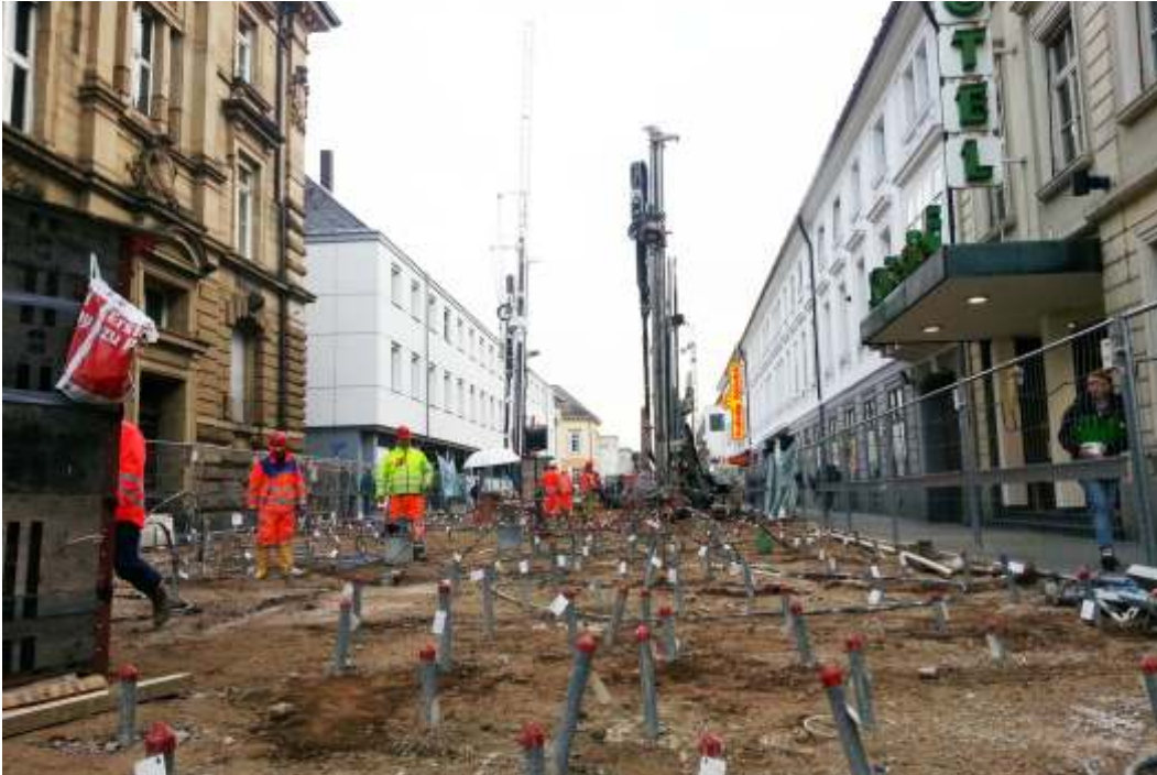
Drilling and grouting works in the Karl-Friedrich-Street
